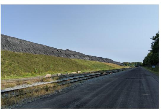
Rio Tinto Fer et Titane (RTFT) P84 dry tailings located in Québec | Partially remediated active TSF dry stack
